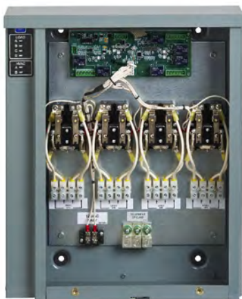
LCM with Terminal Block Connections
